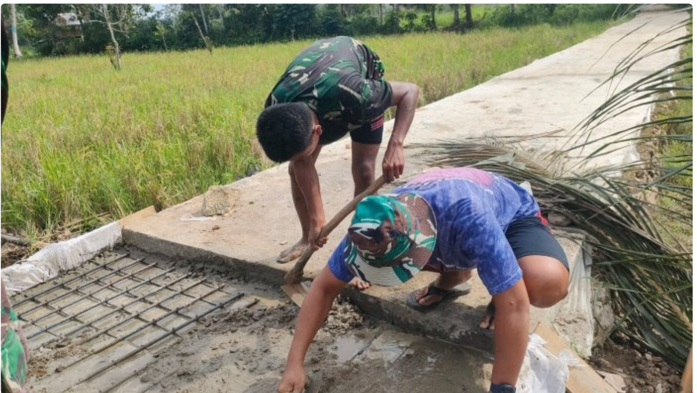
Slop Beton 1 Sasaran TMMMD 116 Kodim 1002/HST Capai 60 Persen
